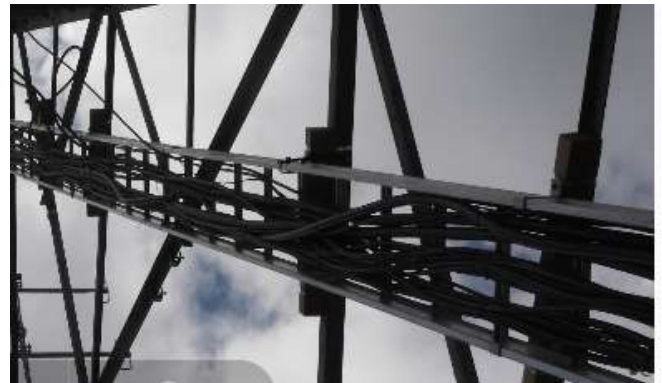
New tray attached to struts with wooden blocks
